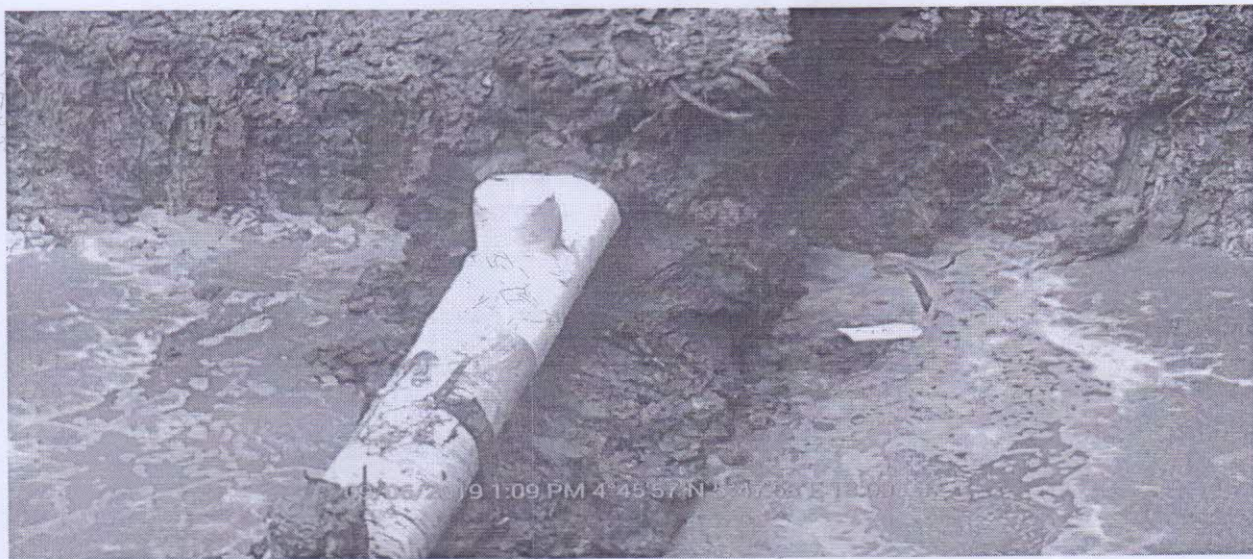
Figure 2: Repair and Wrap Point.
